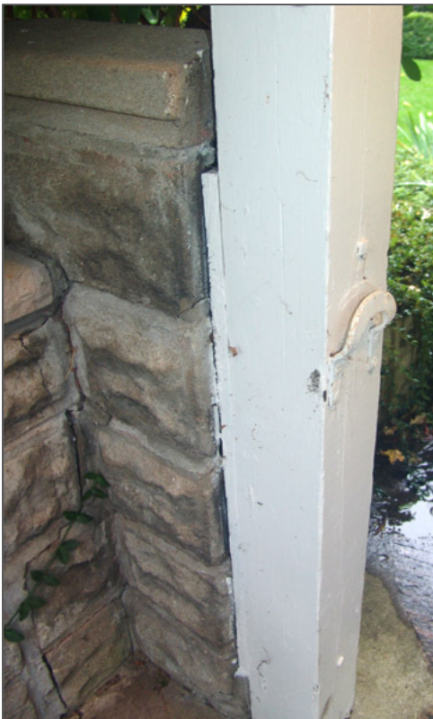
Below Right: Hardware for gate on south support post of pergola
