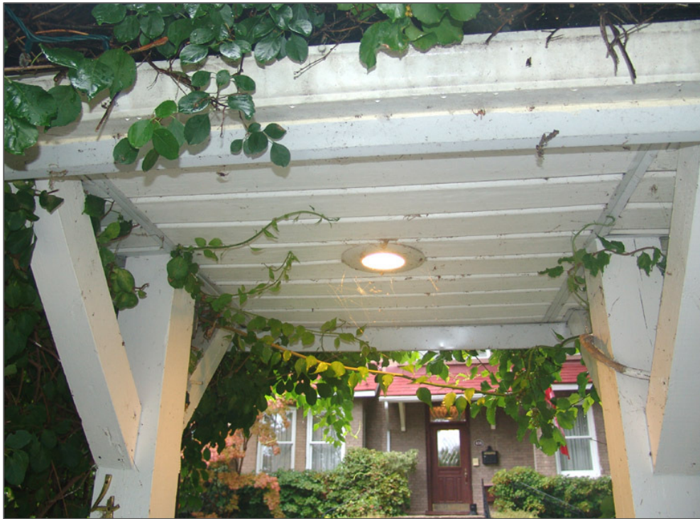
Above: Roof structure, Y-brackets, and support posts of pergola
